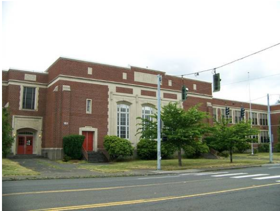
Main building (286A), east (front) elevation, looking west.
