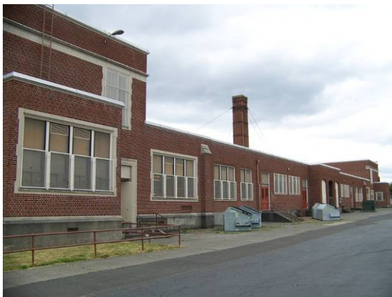
Main building (286A), west (rear) elevation, looking southeast.
