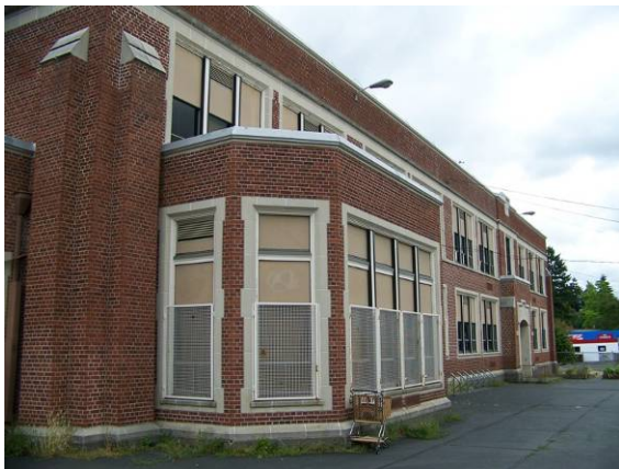
Main building (286A), south (side) elevation, looking northeast.
