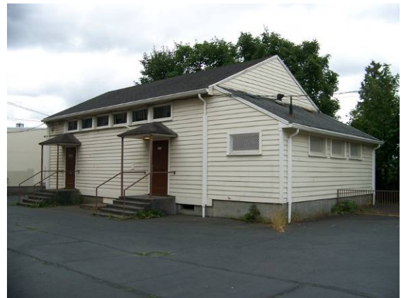
Portable building (No.2), north and west elevations, looking southeast.
